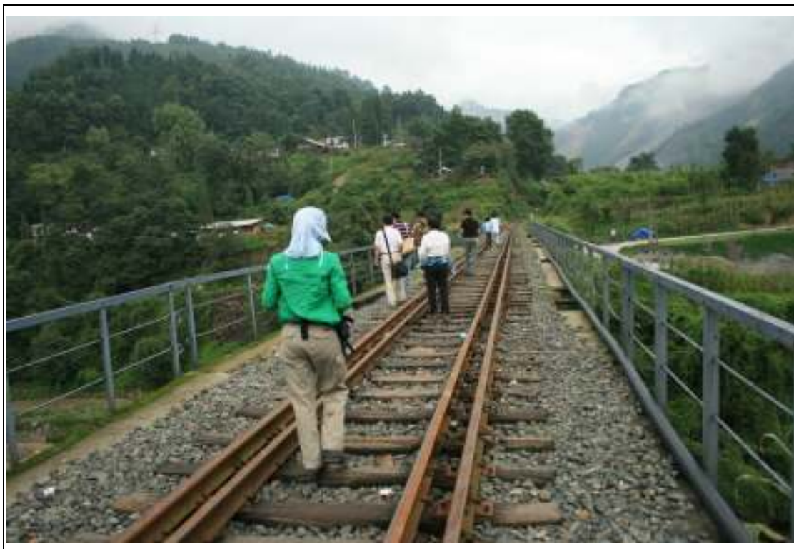
D9: Due to the railway track at 紅白鎮 (Hong Bai Town) was damaged, walking to the landslips & faulted areas about 2km from the road was the only alternative
