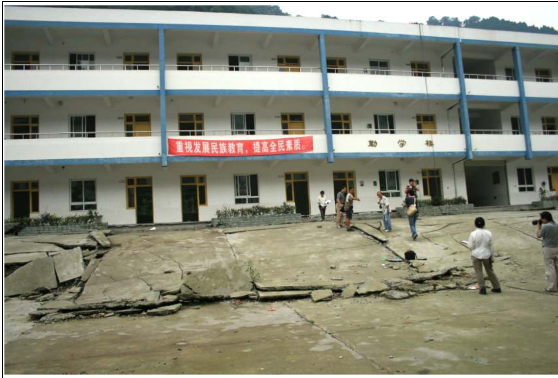
C23: The front view of the school building on the up-thrown side of the fault. This is type-locality of a sinistral reverse-fault caused by the earthquake. It had produced a vertical displacement of 2.2m to 2.3m and sinistrally displaced 4m at the school site.
