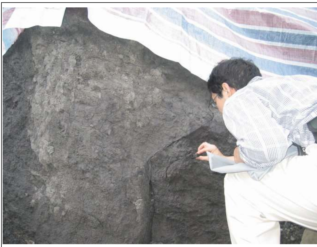
B31: Coal-bearing altered shale where slickensides were observed at 八角廟. The surface rupture was the result of an uplift of ground caused by the earthquake.
