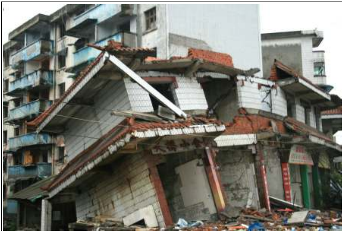
D6: The restaurant at (漢旺) could not escape the from being collapsed.
