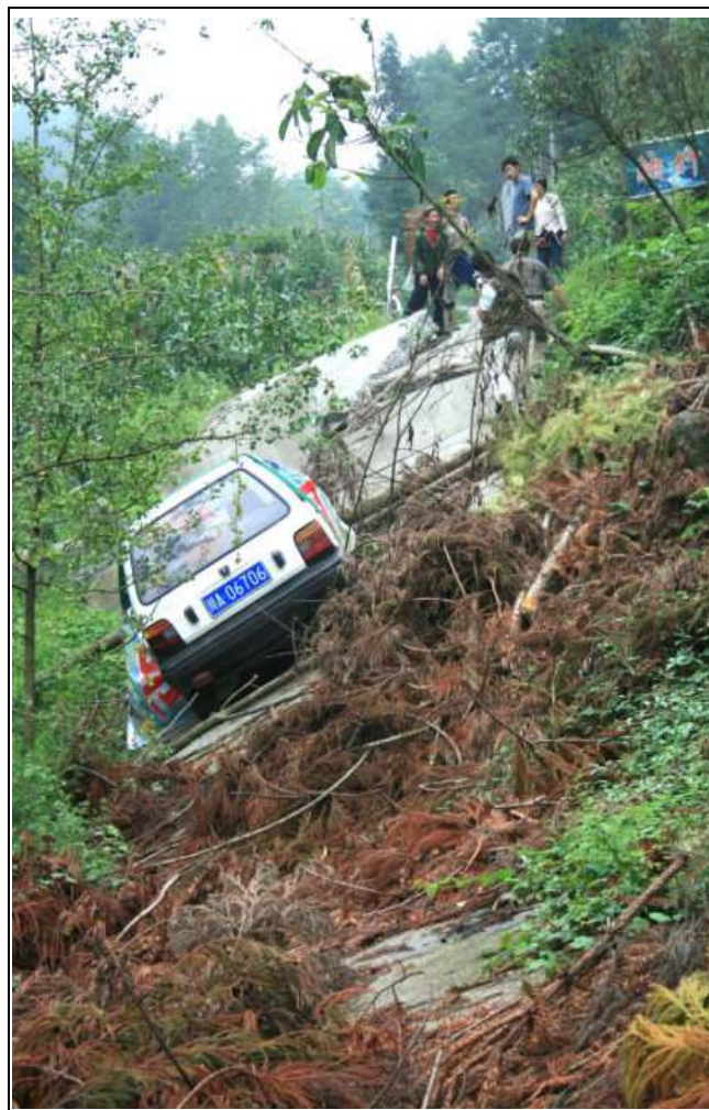
B47: 深溪溝 (Shenxigou) - The degree of tilting of the road was great making it not possible to walk through.
