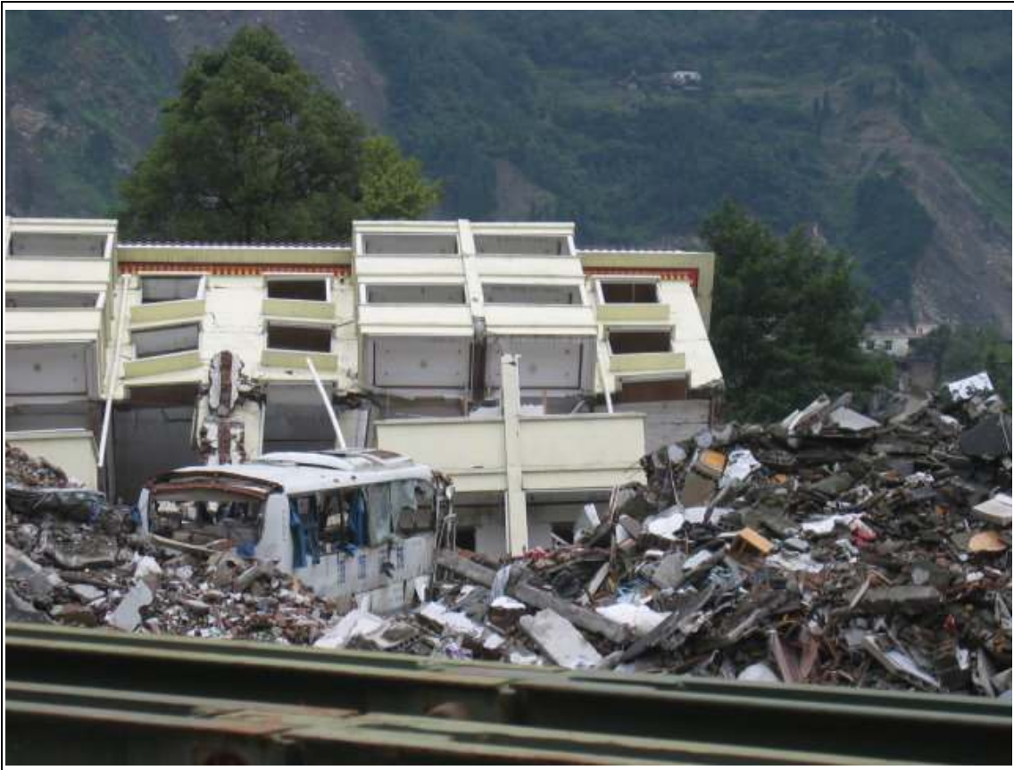
B28: Collapsed buildings and houses were readily captured through camera lens in 映秀 Town
