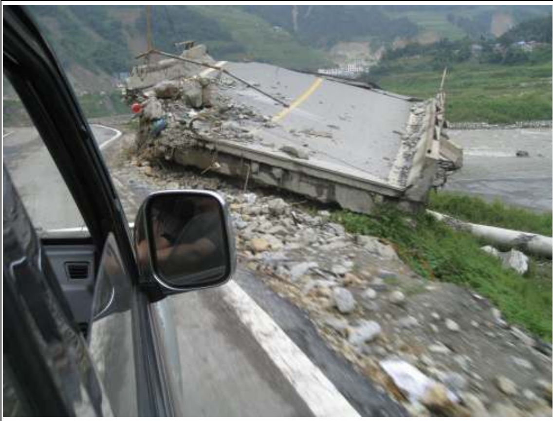
B4a: A highway bridge (白花大橋) was collapsed during the earthquake. The bridge deck was lying flat to ground.
