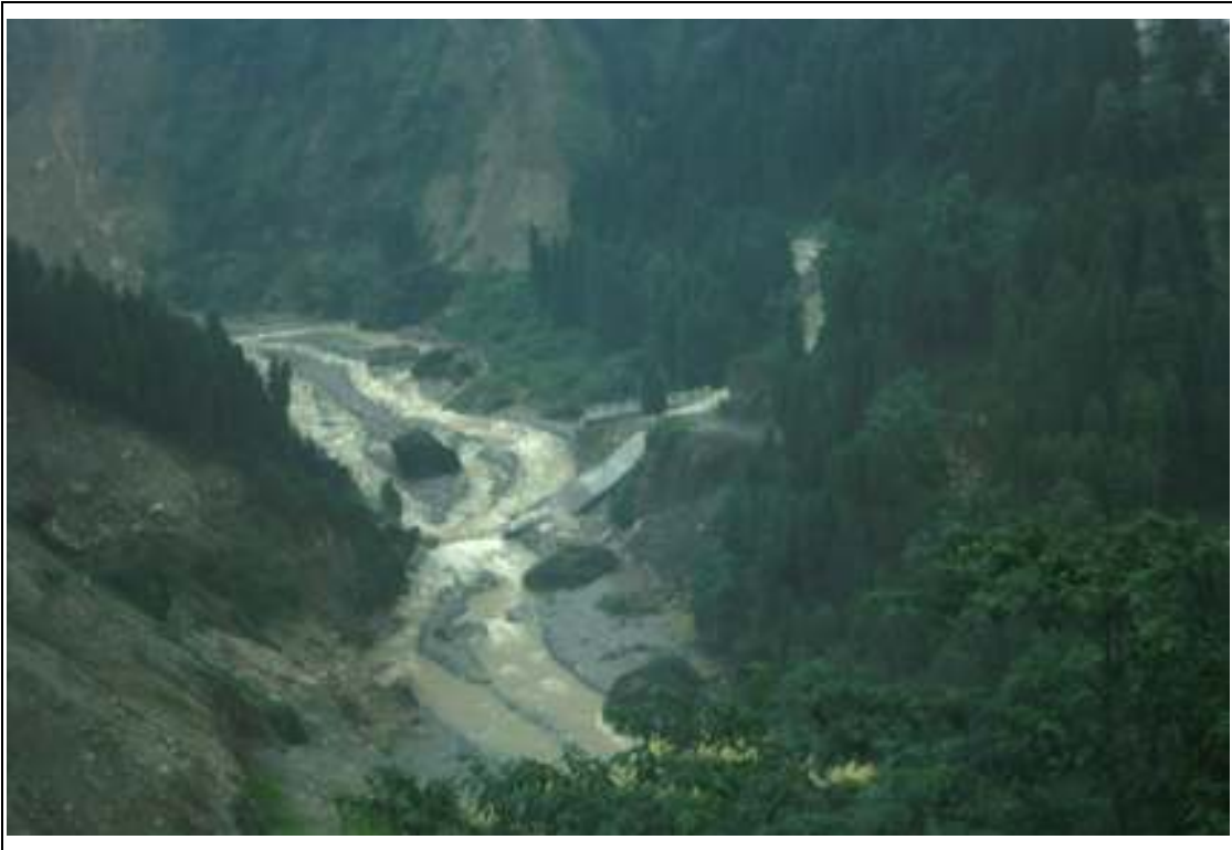
C18: A collapsed bridge was found in the river at 深溪溝 (Shenxigou).
