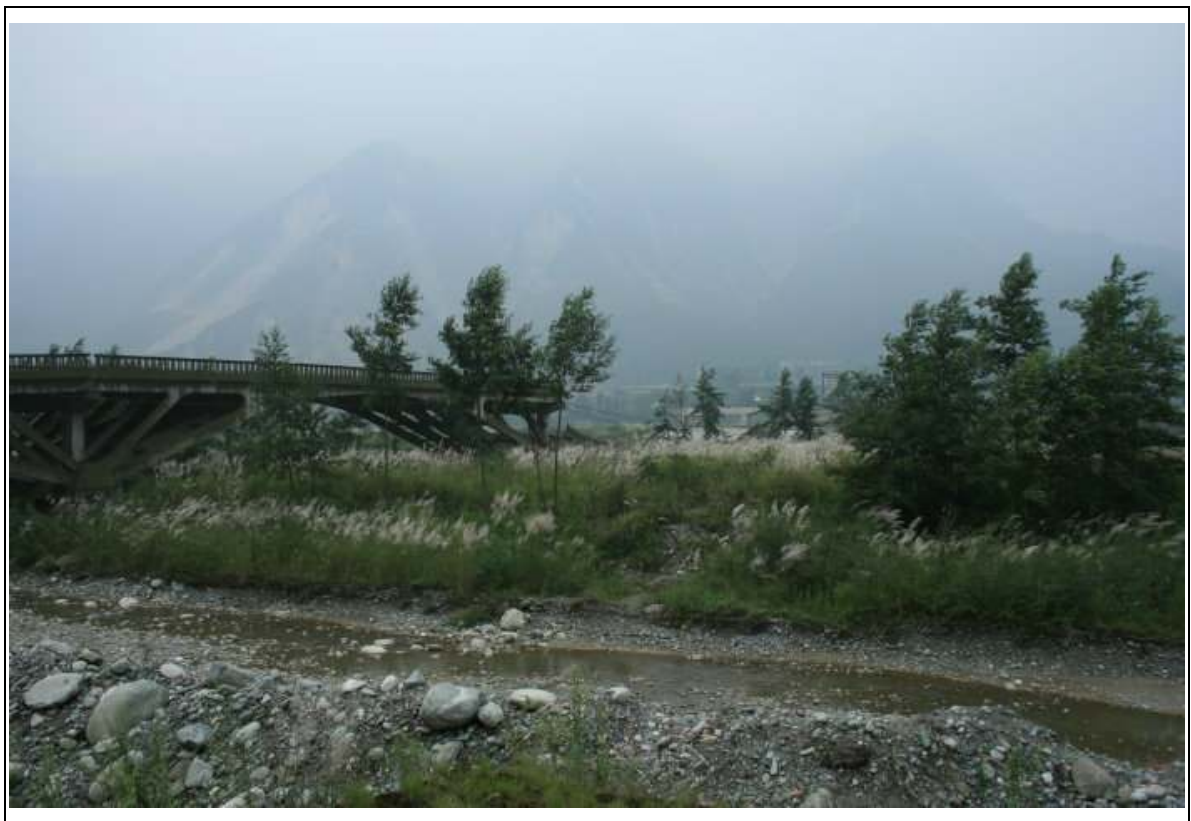
C7: The broken highway bridge viewed from a distance - 小魚洞大橋
