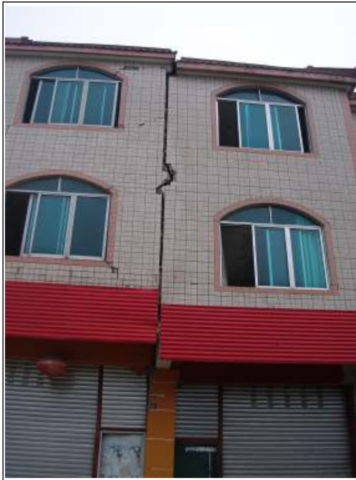
C11b: 小魚洞鎮 – Damaged houses.
