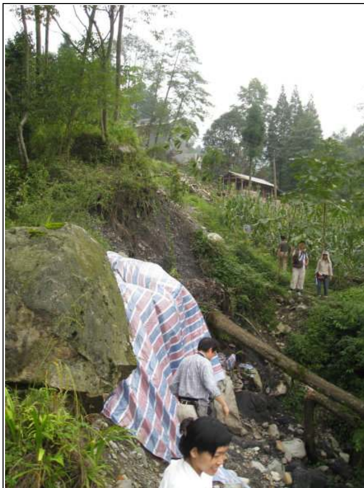
B30: a surface rupture of coal-bearing shale was observed on a slip scar covered by a tarpaulin sheets to protect it from weathering for inspection
