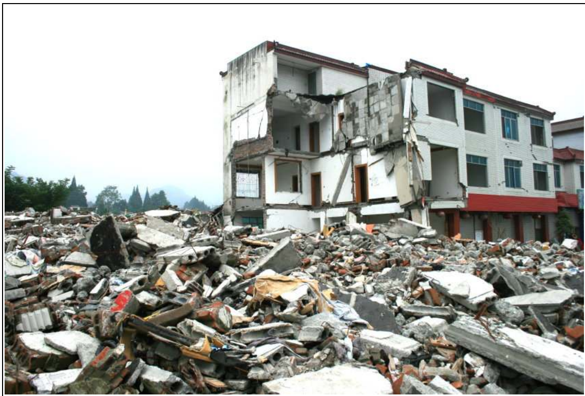
C12: The wreckage of houses indicated that the fault passed underneath them.
