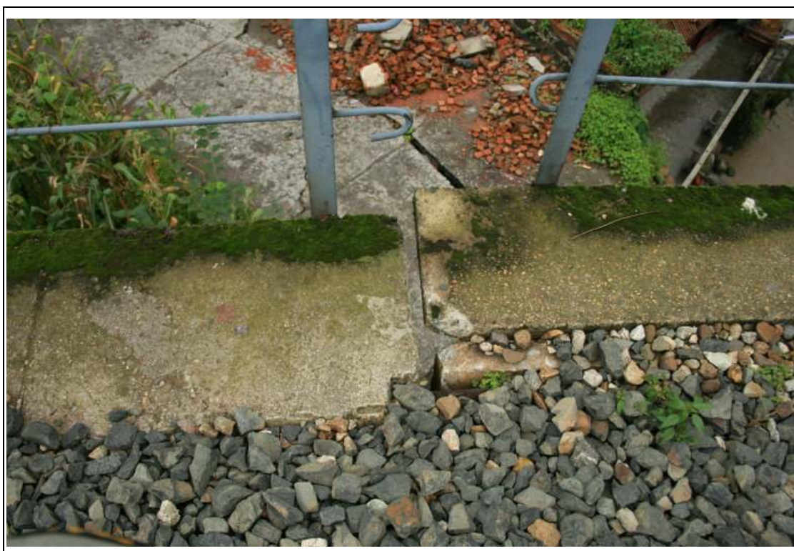
D10: 紅白鎮 (Hong Bai Town) - The railway bridge was also damaged.
