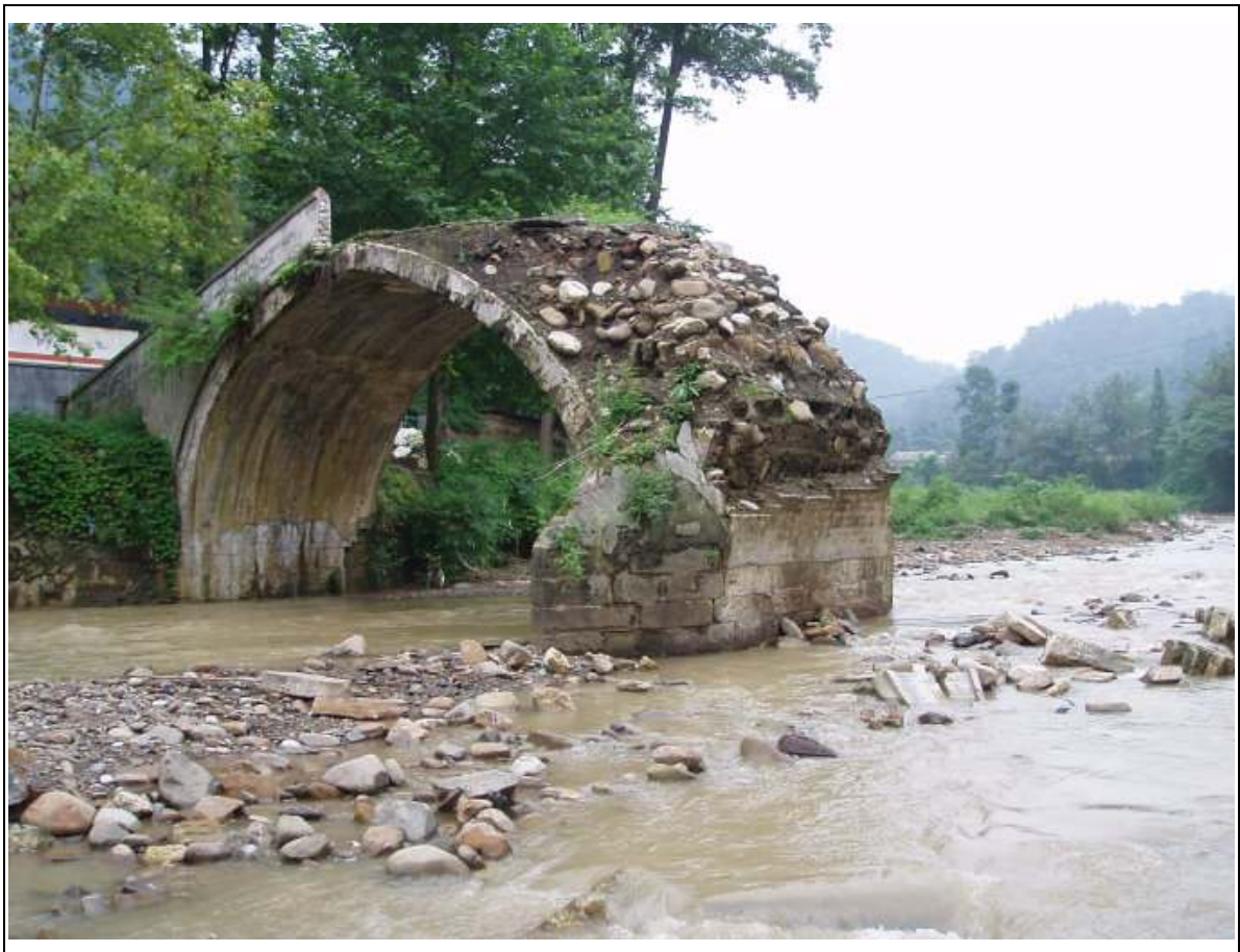
C22a: The Sino-French Bridge near the 白鹿中学校 built as an access to the school across a river was collapsed during the earthquake. The local villagers had then erected their own temporary bridge by putting 7 thick bamboos together across the river.
