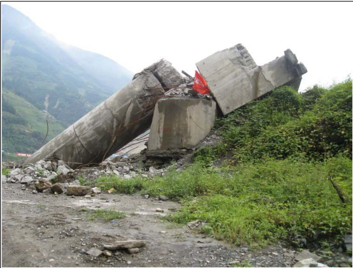
B7: 白花大桥 was down with broken columns and pier of the highway bridge on the verge of the river (白水河).
