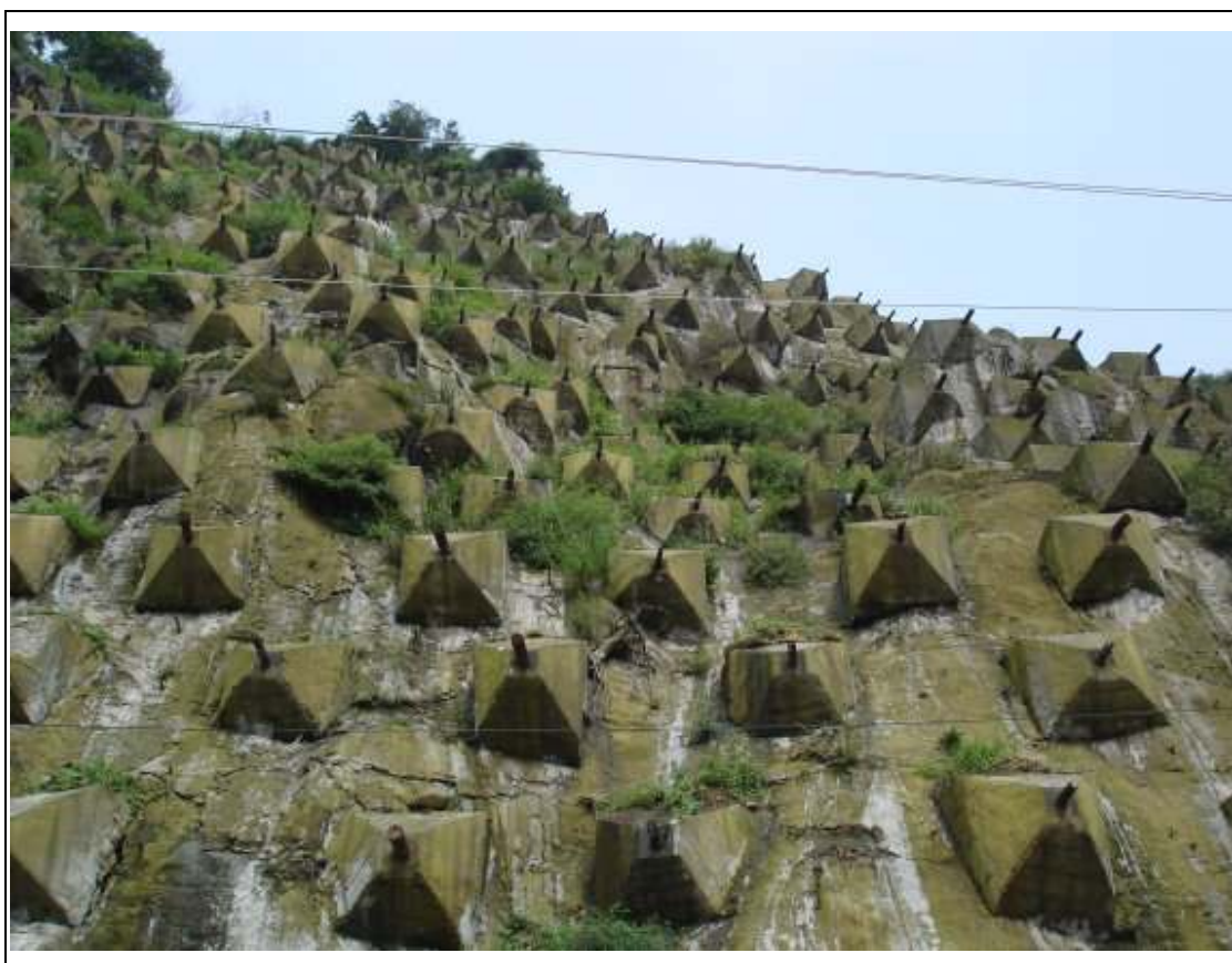
B35: Close-up photograph of rock bolts installed at the dams of the 紫坪壩大橋.
