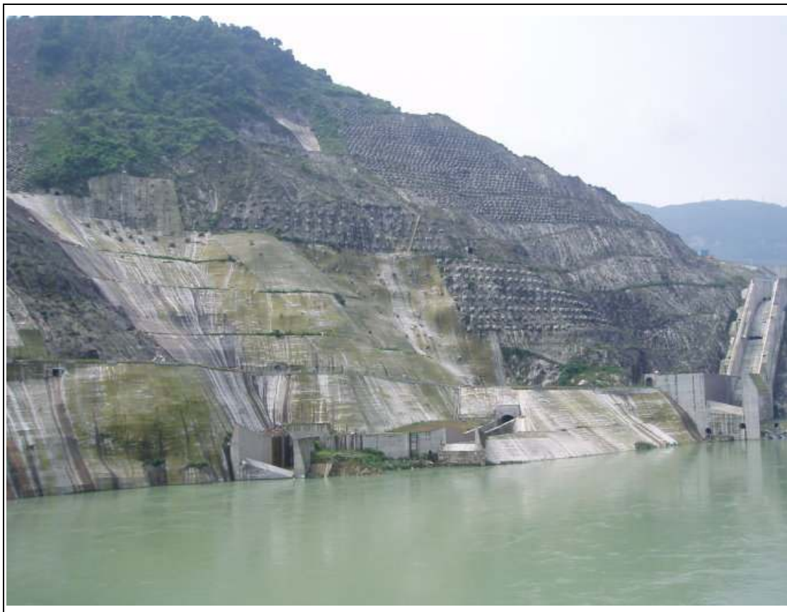
B34: Numerous rock bolts were planted on slope next to the main dam of 紫坪壩大橋 had proved that the dam had resisted the earthquake of such great magnitude.
