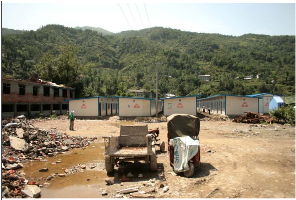
E3: Construction of prefabricated houses for the villagers
