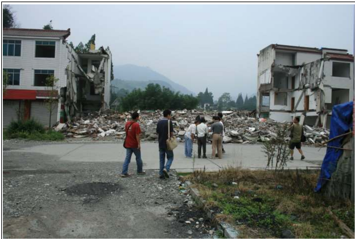
C10: 小魚洞鎮 - The collapsed houses were the footprints of the earthquake.
