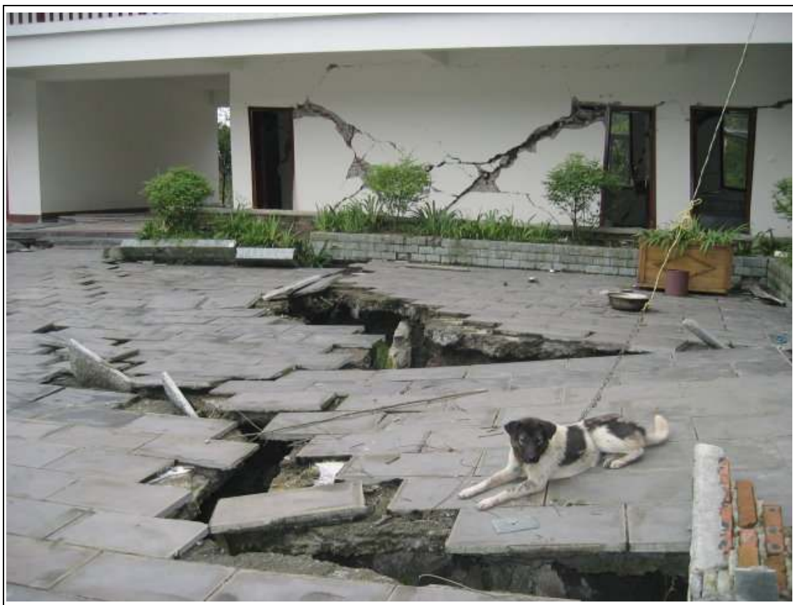
B37: 解放軍訓練中心 (PRC Army Training Centre) at 紅口鎮 - The dog still survived between tension cracks
