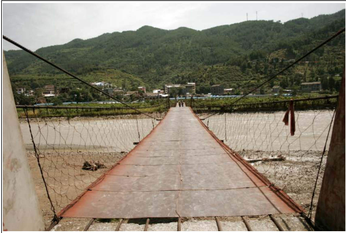
E4 Local people used this simple suspension bridge as access to the opposite side of the river.
