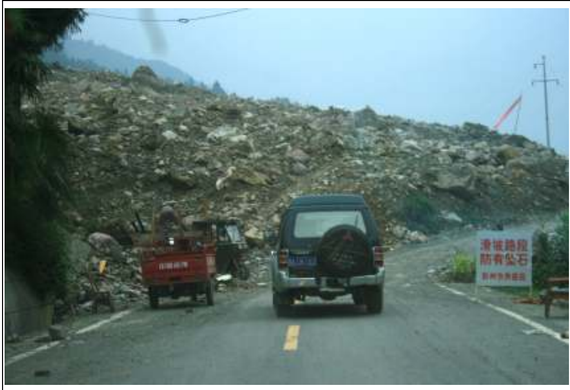
C20: Large quantity of debris could be seen from the road at 深溪溝
