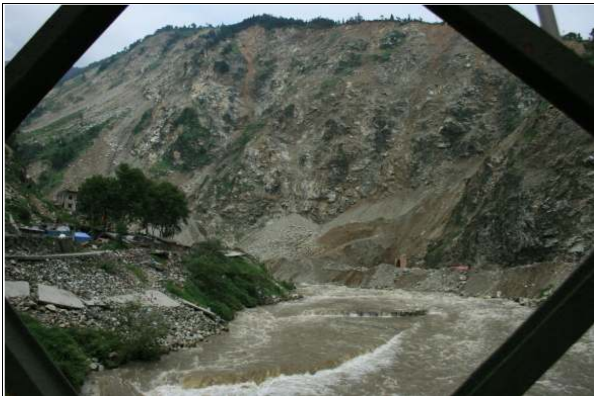
B26_The mountain was totally stripped off and the river bed was disrupted in 映秀 Town. 百慈大橋 was collapsed. A temporary steel bridge was erected for the transportation of daily needs to the villagers.
