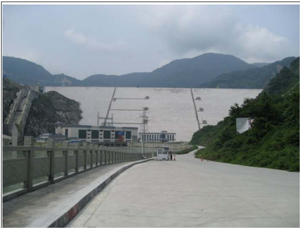
B33: 紫坪壩大橋_Main dam was reported to have no significant damages
