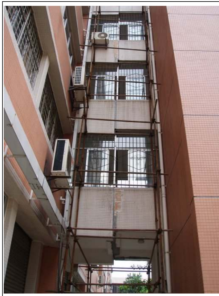
A6: Building within the campus of Sichuan University was damaged.
