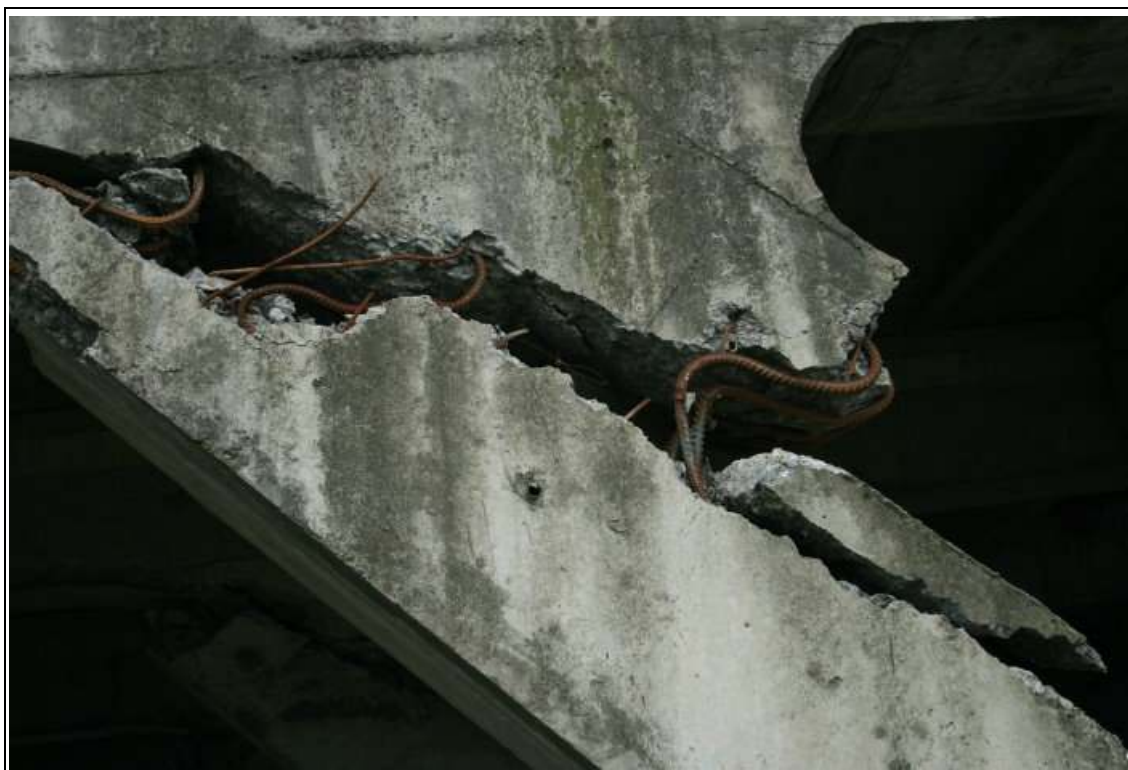
C6: Distorted reinforcement of the 小魚洞大橋
