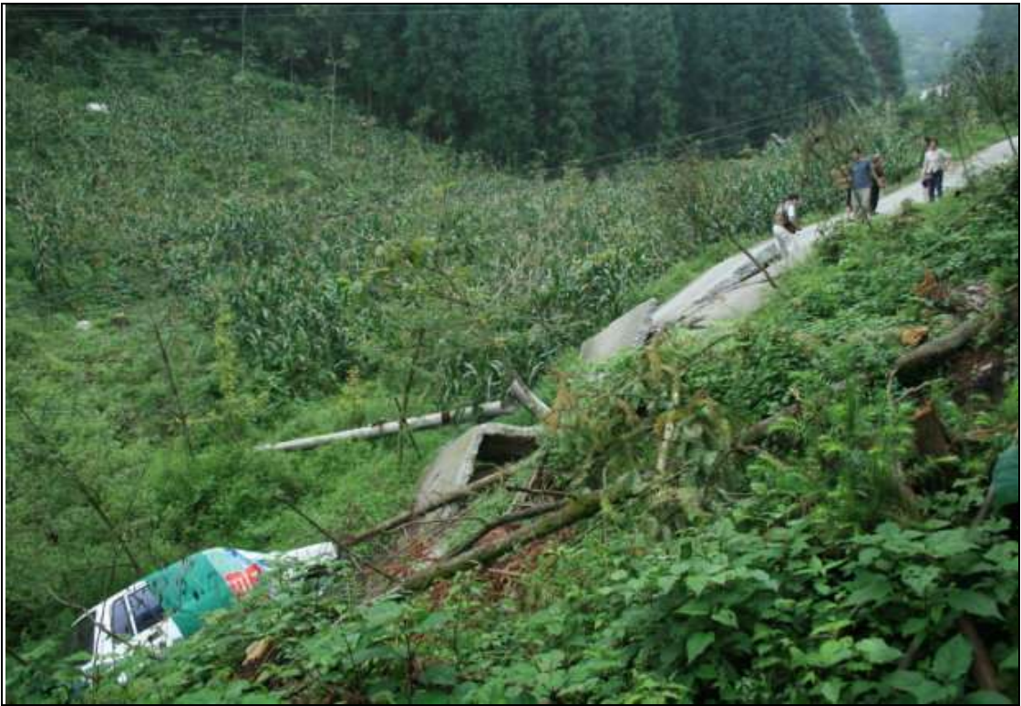
B46: 深溪溝 (Shenxigou) - The access road to villages in the mountain was tilted and “buckled”.
