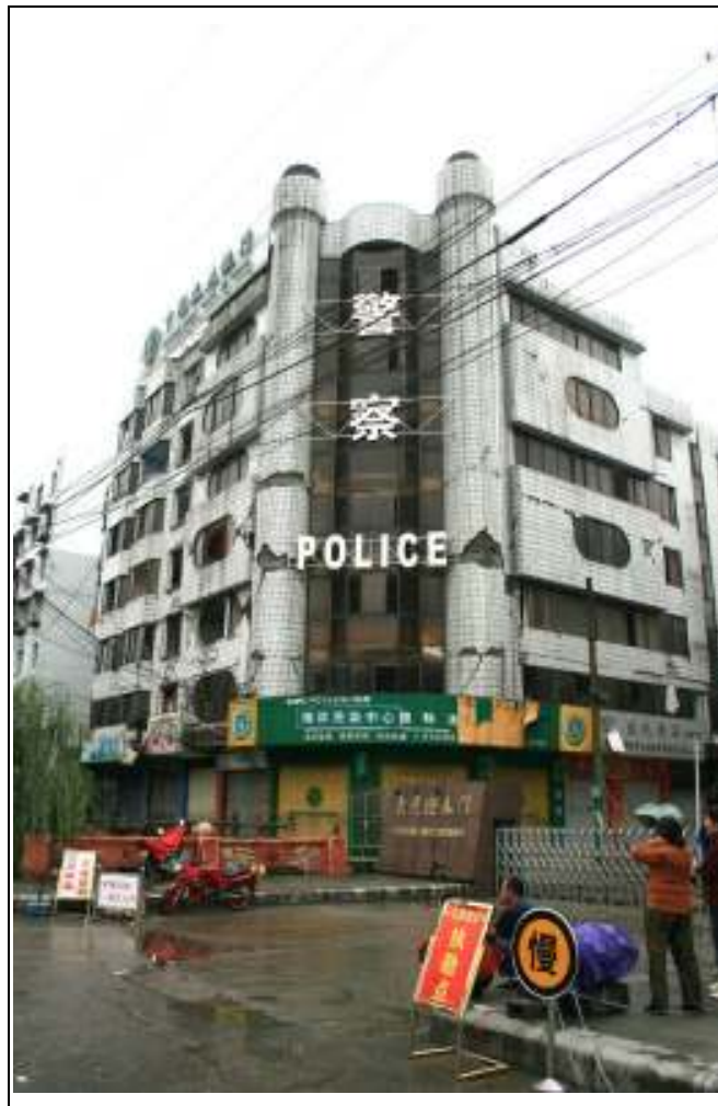
D5: The police office at Hon Wang (漢旺) was also damaged.
