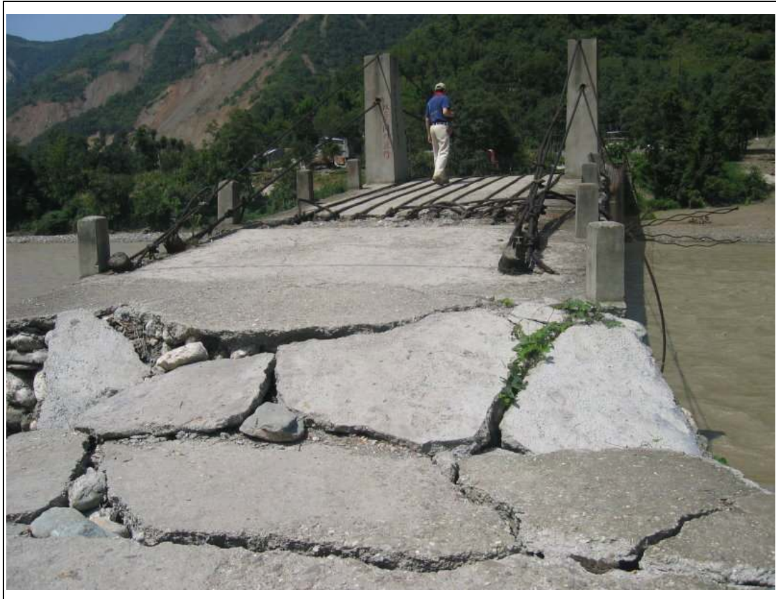
E4a: During the earthquake, part of the bridge was damaged.
