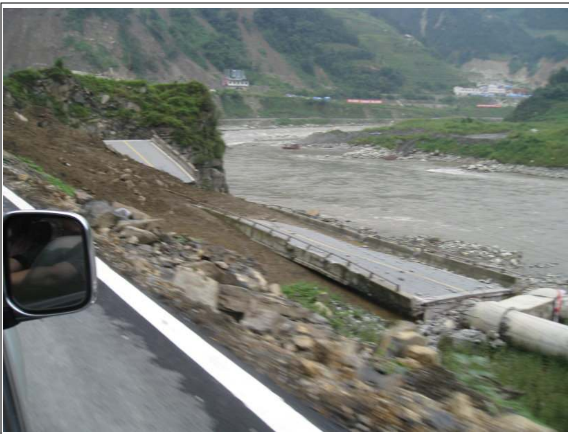
B5: The collapsed deck and columns of the highway bridge (白花大橋) were detached (adjacent to 白水河).
