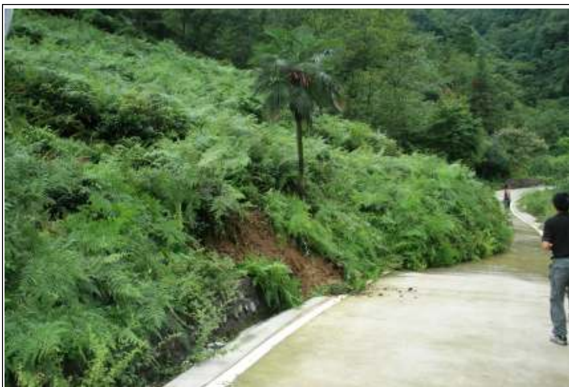
D14: 金花镇 (Jin Hua Town) - A landslide noted at mid-level of mountain.
