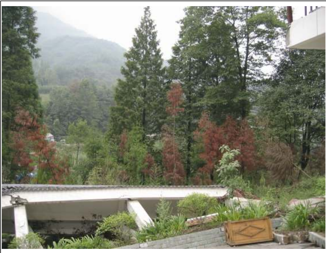
B39: 解放軍訓練中心 (PRC Army Training Centre) at 紅口鎮 - The trees adjacent to the fault disruption were wilted with brown colour, other trees unaffected remained green.
