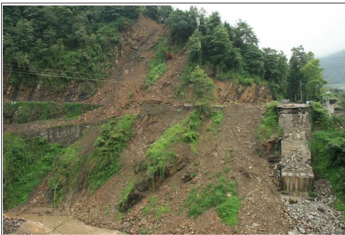
D8: At 紅白鎮 (Hong Bai Town), a road bridge across a river was collapsed and the access to the opposite side of the town was hampered.
