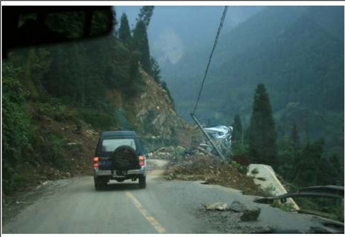
C19: On the way to 深溪溝 (Shenxigou), highways were often blocked by landslips and part of the road had been fallen into the gorge.
