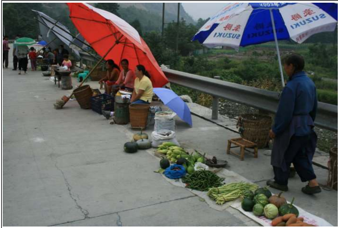
C9: 小魚洞鎮 - Villagers moved their market to the damaged bridge at 小魚洞大橋 in order to earn for a living.
