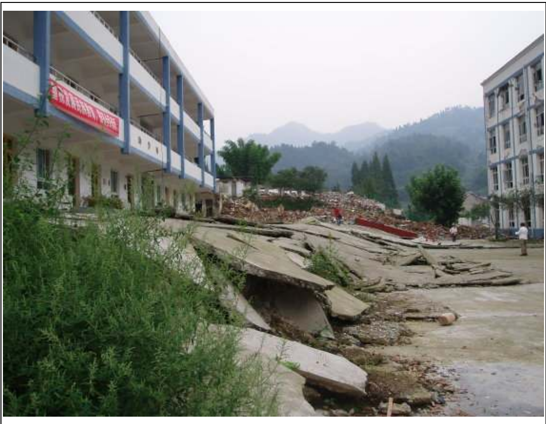
C25: The upthrown side of the school remained intact whereas the school at the downthrown side was slightly damaged
