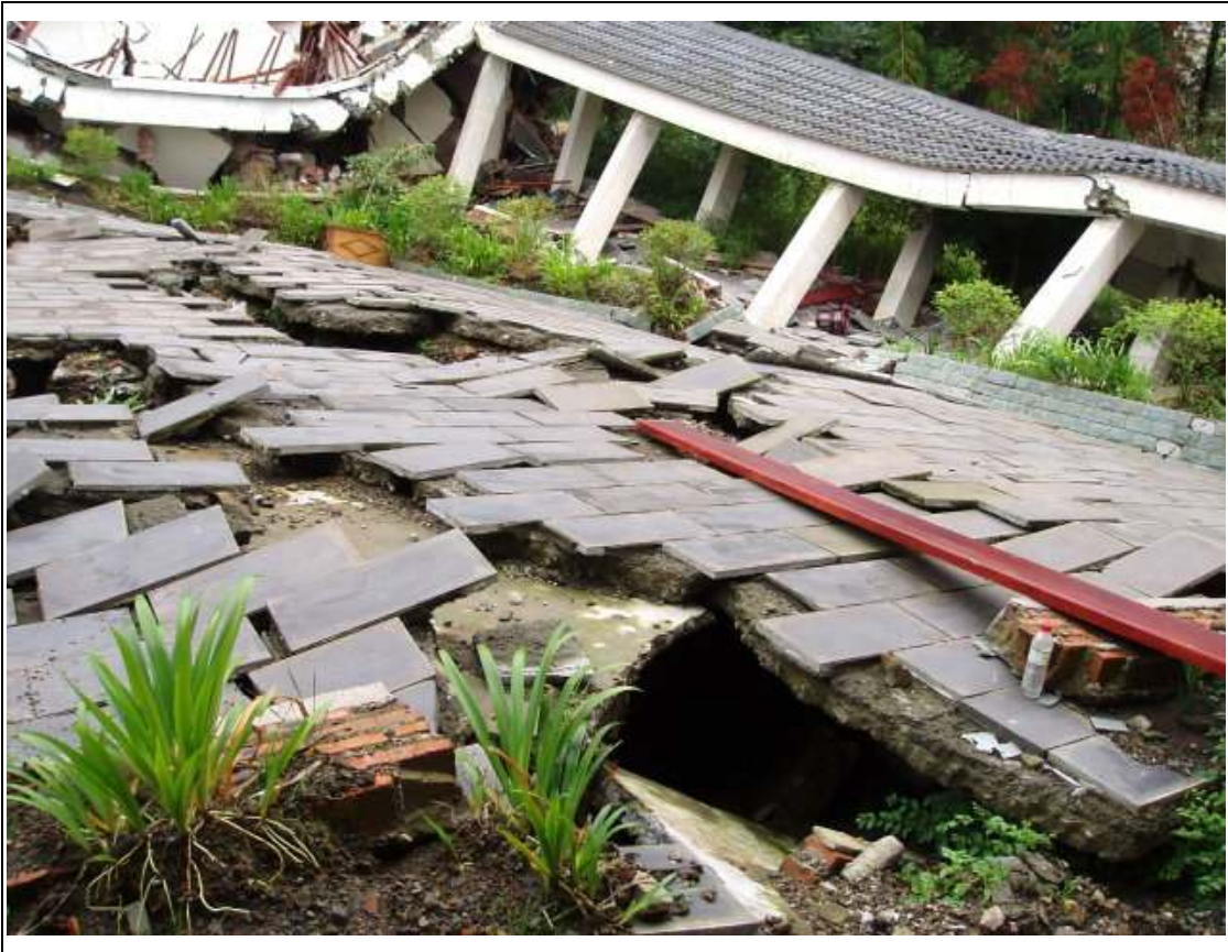
B38: 解放軍訓練中心 (PRC Army Training Centre) at 紅口鎮 - The structure were seriously damaged by the quake leaving behind the wide and deep tension cracks on ground.
