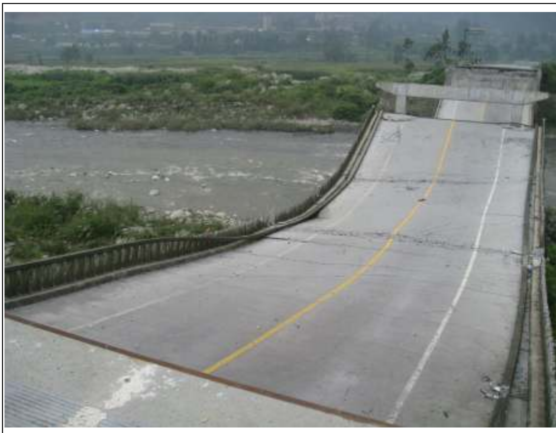
C5: The highway bridge.(小魚洞大橋) was collapsed into several sections, the bridge columns were detached, joints dislocated with some of the steel reinforcement distorted and exposed; the road surface of the bridge was cracked and offset.
