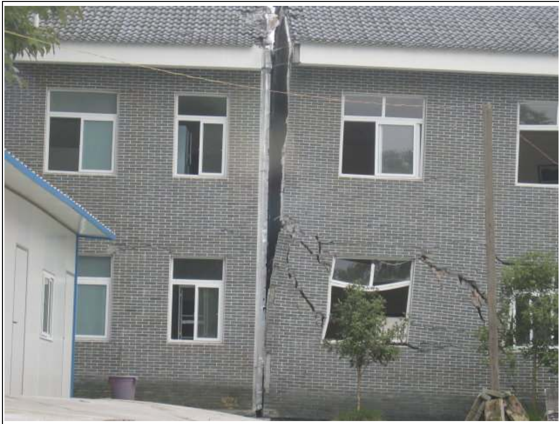
B36: 解放軍訓練中心 (PRC Army Training Centre) at 紅口鎮 - Buildings were detached and shearing stress demonstrated notably near windows.
